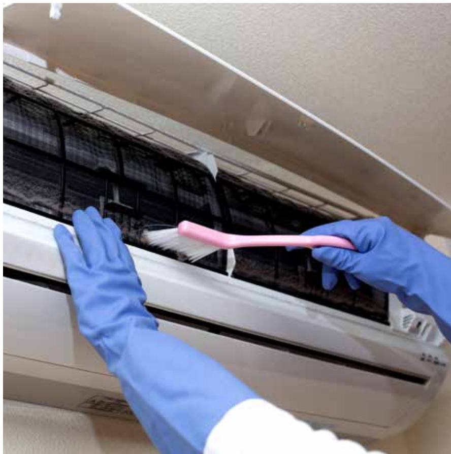
► Regular preventive maintenance of AC units is required to increase the efficiency of the system
